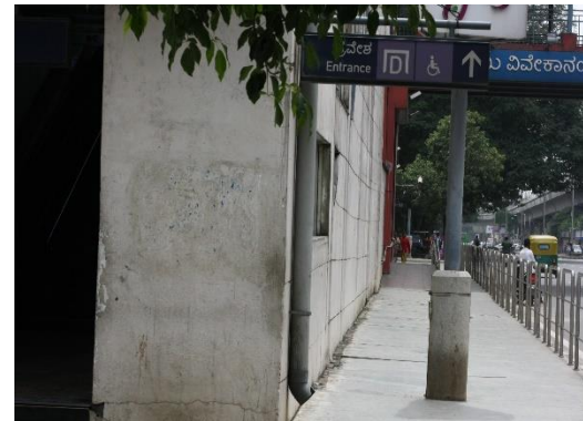
Figure 50: Signage at access point C
