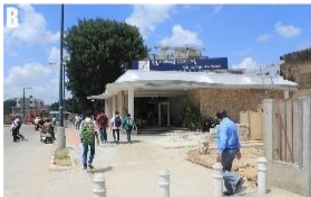
Figure 59: Access point B
