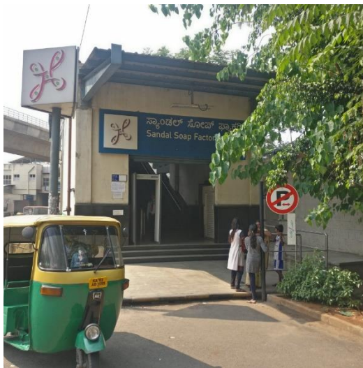
Figure 29: Access point A
