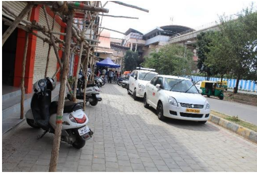
Figure 5: Parking on footpath at access point A
