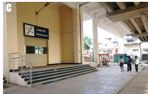
Figure 24: Access point C
