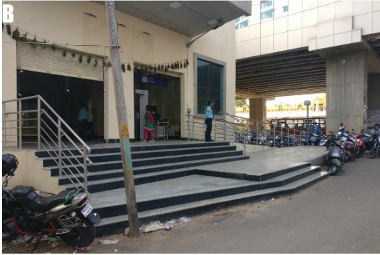
Figure 22: Access point B
