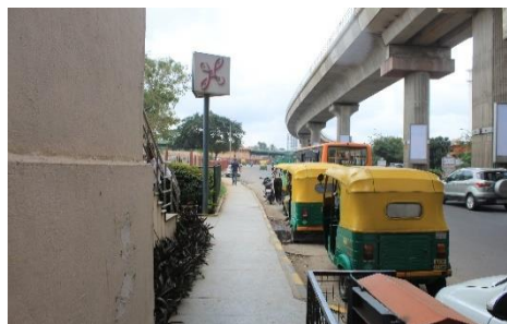
Figure 17: Footpath at access point G
