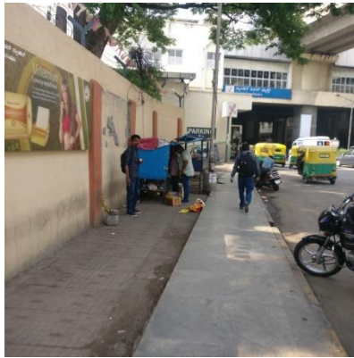
Figure 32: Footpath at access point B
