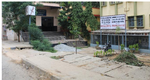
Figure 10: Footpath at access point C
