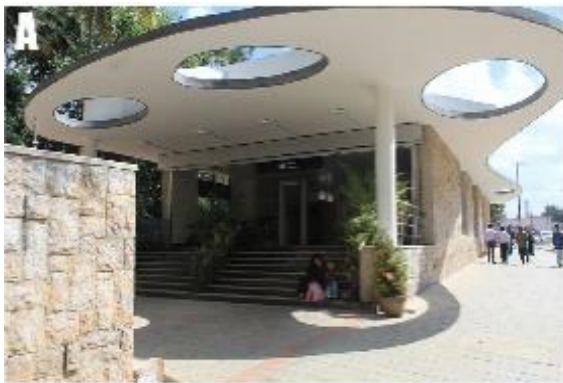
Figure 57: Access point A
