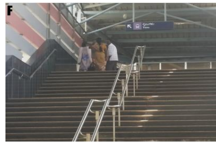
Figure 15: Staircase at access point F
