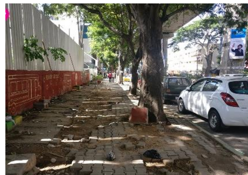
Figure 43: Footpath at access point C
