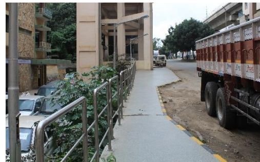
Figure 8: Footpath at access point B
