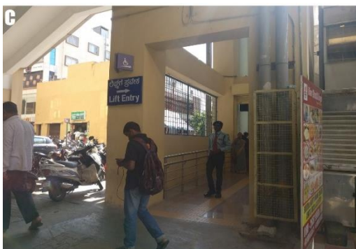
Figure 42: Access point C
