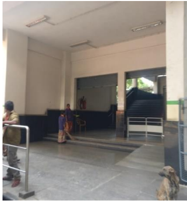
Figure 31: Access point B
