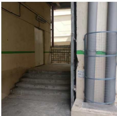
Figure 34: Access point C
