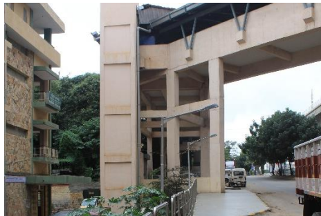
Figure 7: Access point B
