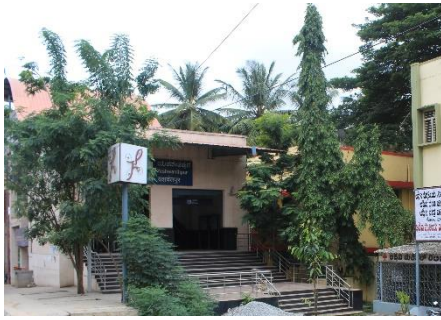
Figure 9: Access point C
