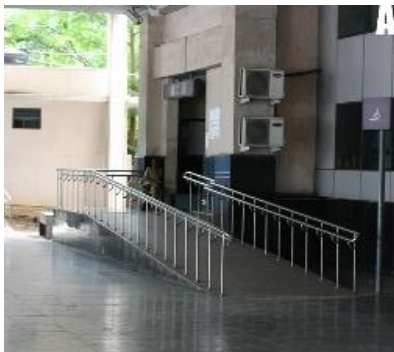
Figure 46: Access point A
