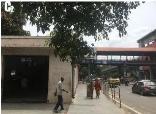
Figure 49: Access point C
